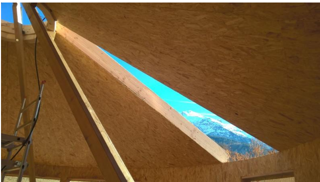
Roof panel construction
